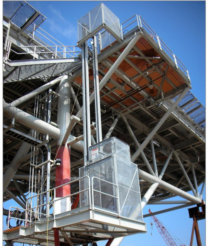
Guide columns are 6" wide flange sections. The carriage is fabricated of 4" or 6" structural members with a steel deck plate. Additional deck surfaces are available.
